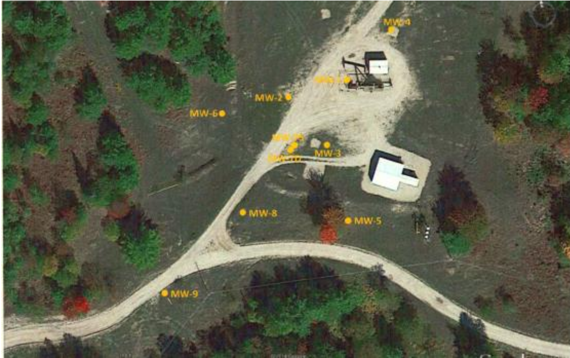
Monitoring Wells on Site
